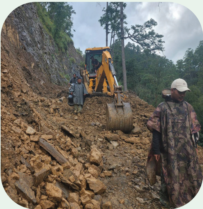
Road maintainance in Chinland
